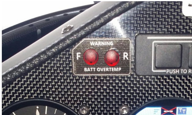
Battery overtemperature warning lights
